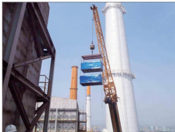
**Figure 1.** Installation of the KIST catalyst to the De NO<sub>x</sub> system of POSCO sintering furnace.
